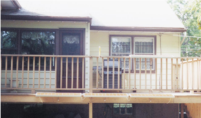
Above: These four PV modules provide power for communications and lighting.
